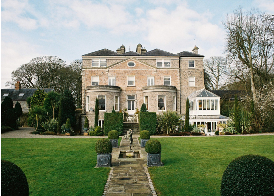
Image 9.2: View of the rear façade of Osberstown House: the bows and the right hand bay are later constructions, as is the conservatory
