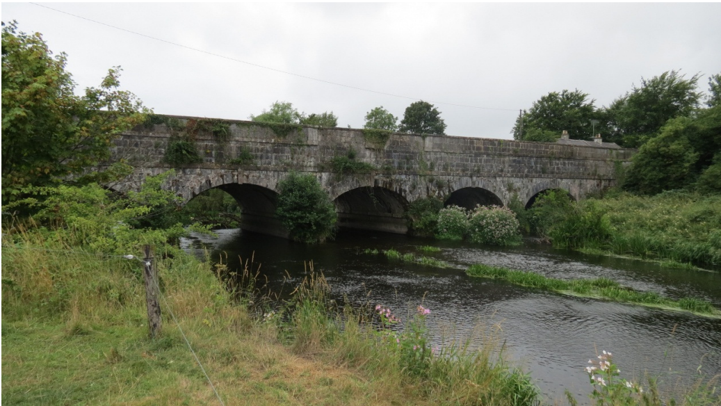
Image 9.12: View of the Leinster Aqueduct from river
