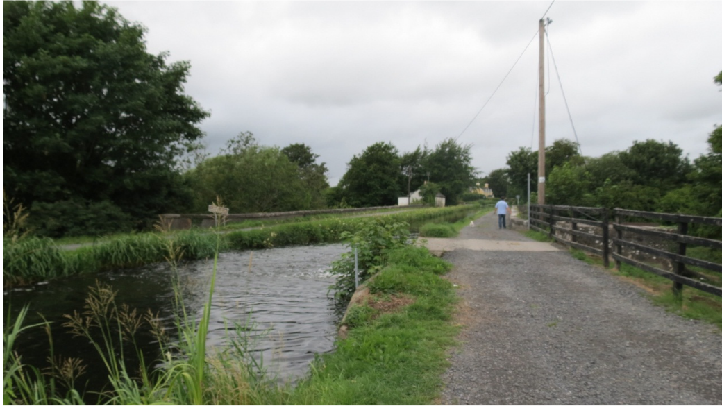
Image 9.13: View along canal at aqueduct
